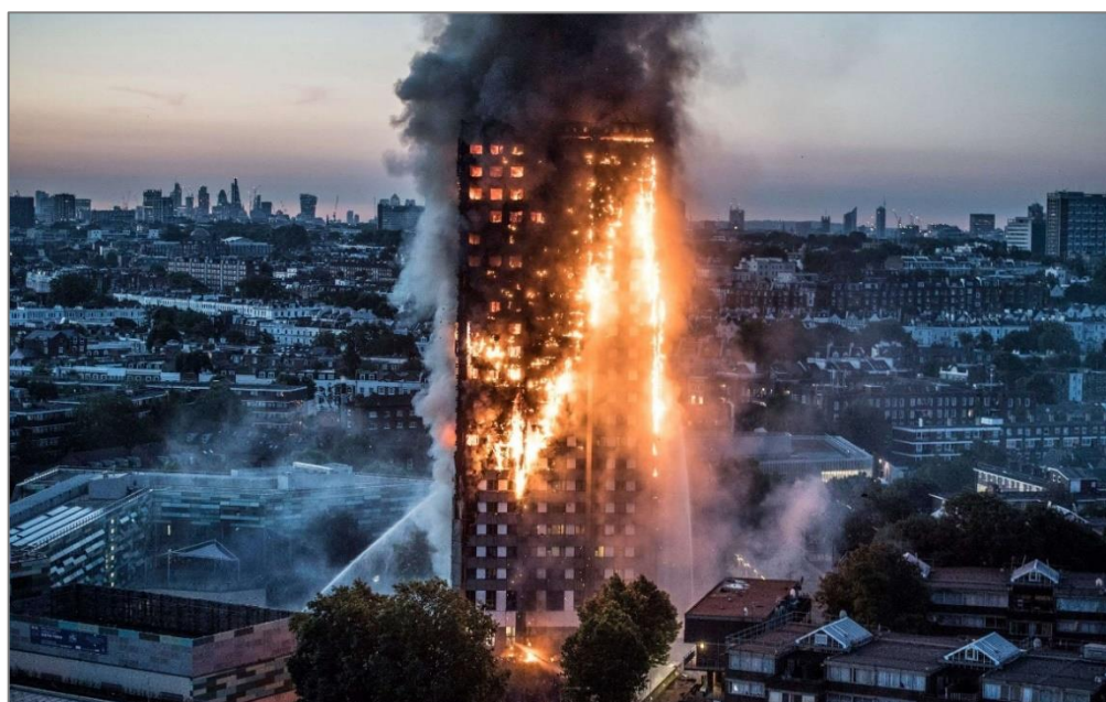
Рис. 1. Пожар в Grenfell Tower 1 Fig. 1. Fire in Grenfell Tower
